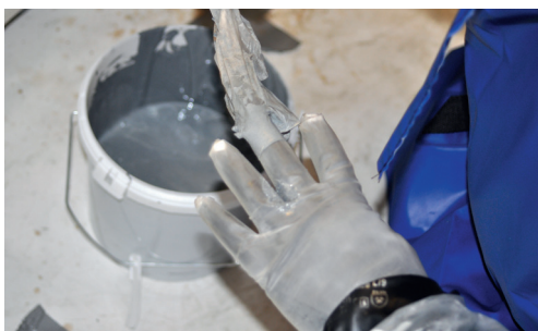
5. The glove is pulled off with one hand and placed in the coating residue.
