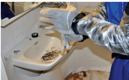
1. To coat the floor drain, long chemical protection gloves are put on first, followed by 2-4 thin vinyl gloves on top of them.
