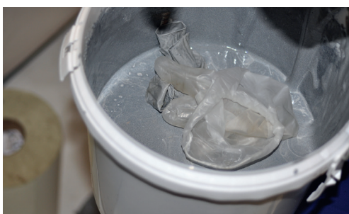
7. The coating residue is left to harden in the bucket and is appropriately disposed of.
